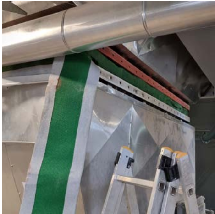
Slika 18. Cementara/ Cement plant
