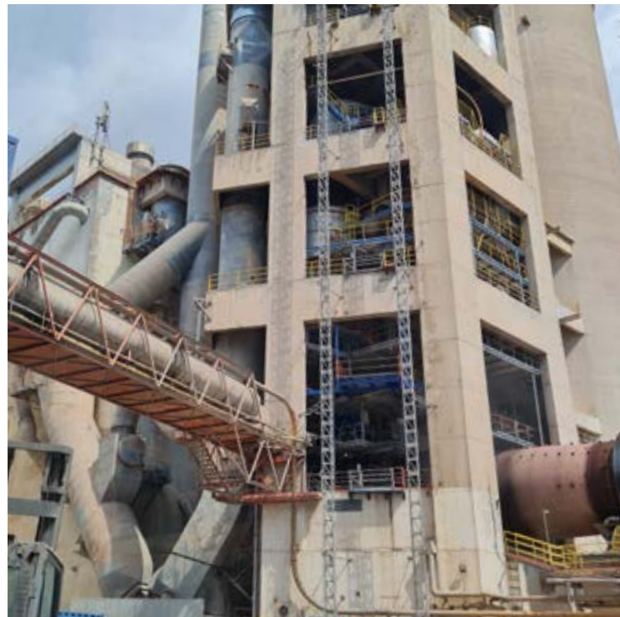
Slika 38. Cementara/ Cement plant
