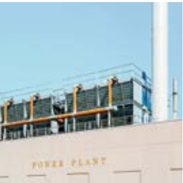
Energane/toplane/ Power plants/heating plants
